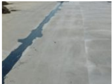
RCC Slab Joint
