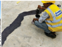
RCC Crack Repair
